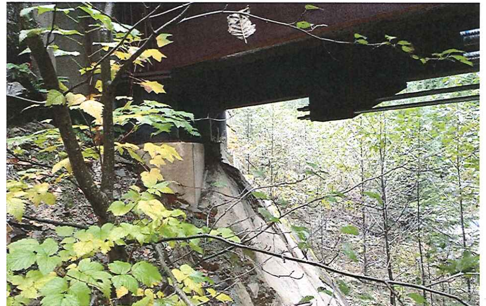
CK2111 Left Abutment
