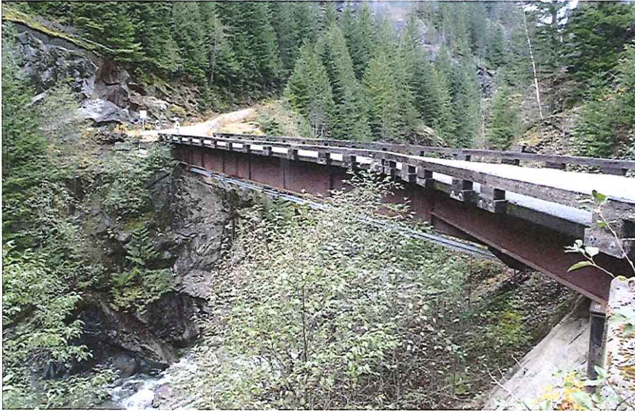
CK2111 From Downstream
