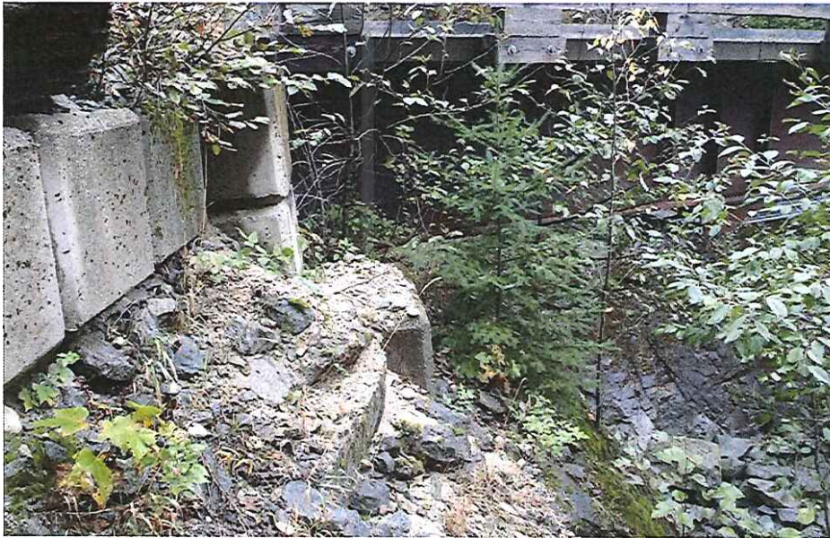
CK2111 Right Abutment
