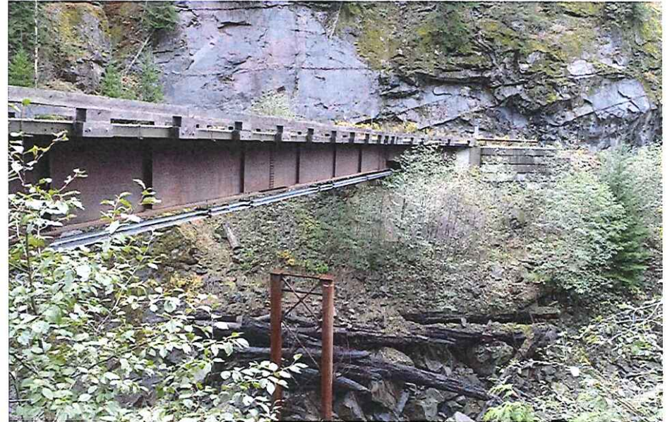
CK2111 From Downstream Right
